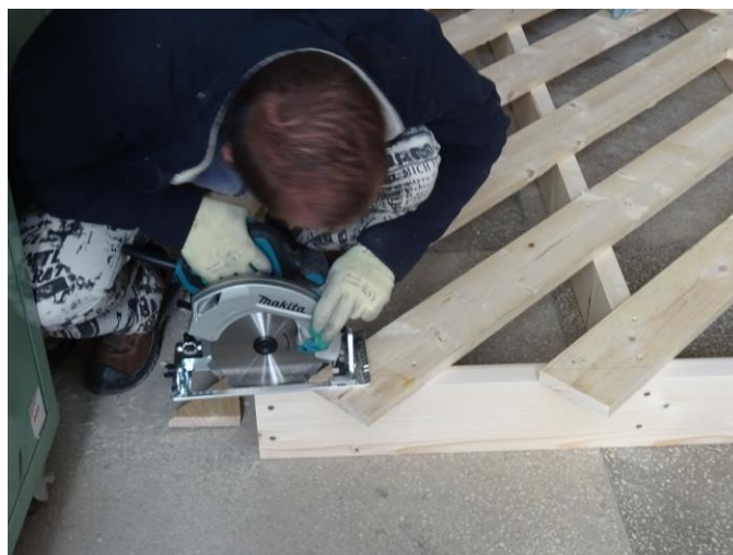
Figure 6 – Cutting the out triggering parts of the timber planks
