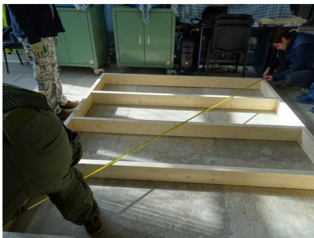
Figure 5 – Execution of the internal structure of the modulated wall
