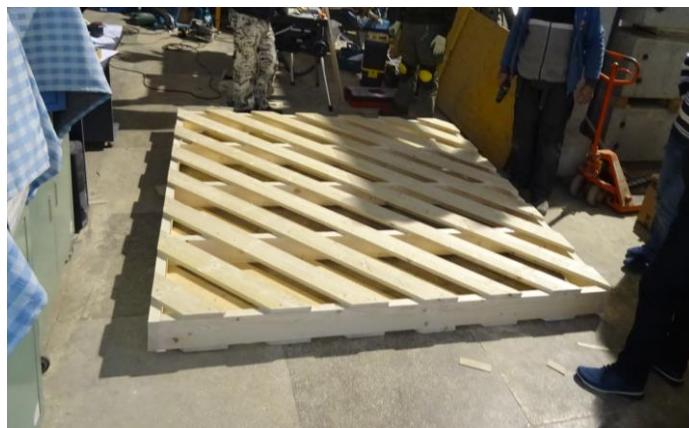
Figure 8 – Applying the timber planks on the other side
