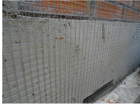
b – mesh applied on the concrete surface and also on the masonry
