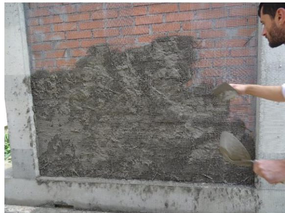
j – the mortar finishing is applied by hand throwing
