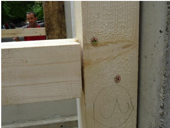
Figure 6. Connection execution error – existing big gap
