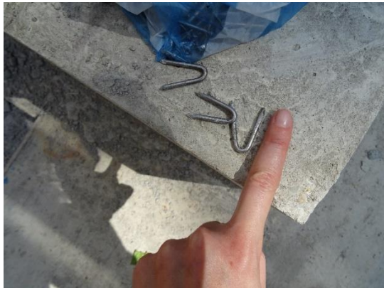
a – nails used to position the wire mesh on the concrete (mesh was at 1 cm distance from the concrete surface)
