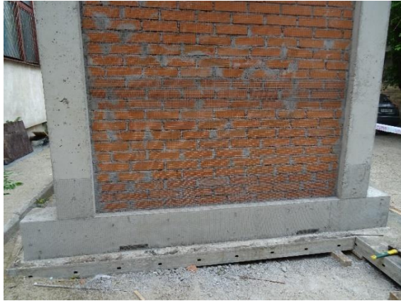
g – overlapping wire mesh from RC beam on the masonry
