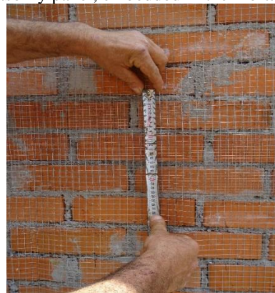
d – the clamps applied to position the wire mesh on the masonry panel, embedded in the mortar joints
