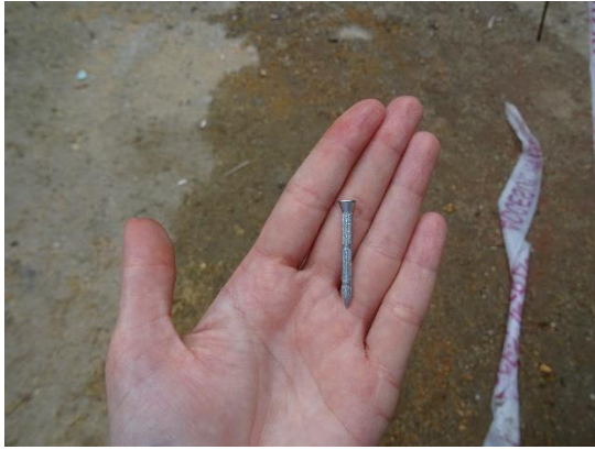
a – nails used to position the wire mesh on the concrete (mesh was at 1 cm distance from the concrete surface)
