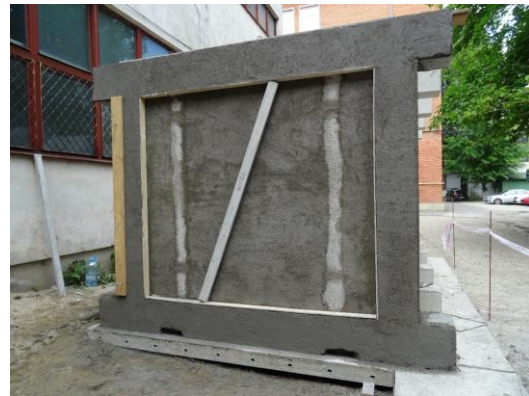
j – the mortar finishing is applied by hand throwing
