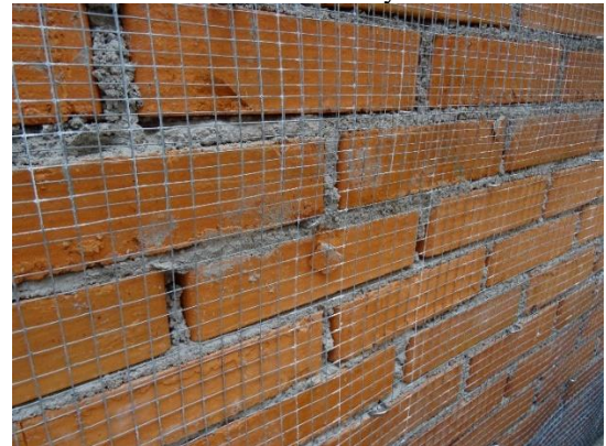
b – mesh applied on the concrete surface and also on the masonry
