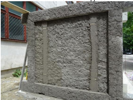
k –starter layers applied for reference thickness of the mortar layer
