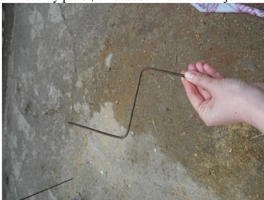
c – the clamps used to position the wire mesh on the masonry panel, embedded in the mortar joints
